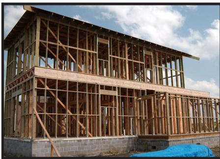
Advanced framing - larger lumber, but wider spacing and stack framing provides strength and more insulation with fewer studs and lower framing cost.
